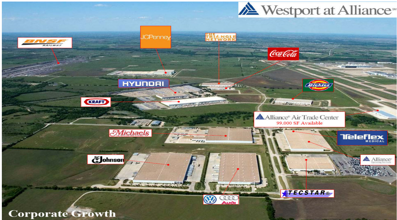
Figure 3.7 Intermodal Logistics Center served by Rail and Airport
